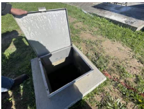
Photo 21: View of the water cistern located on the northwest exterior corner of the nightclub.
