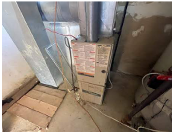
Photo 14: View of one (1) of several natural gas fired furnaces located within the motel.
