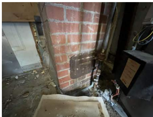
Photo 18: View of the chimney and chimney cleanout centrally located within the motel.
