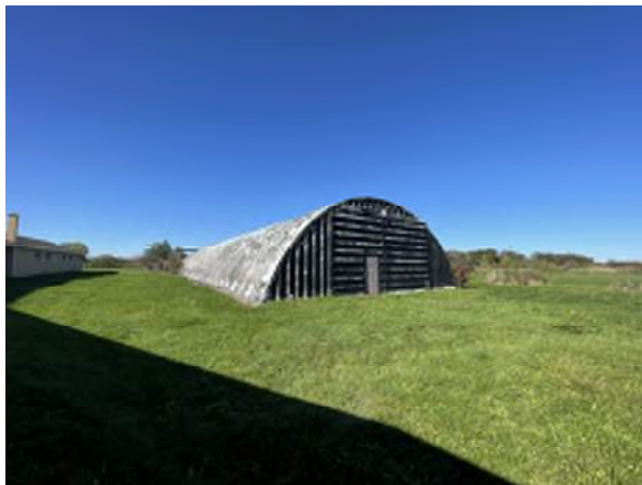
Photo 19: View of the Quonset hut located northwest of the motel. Photograph taken facing west.
