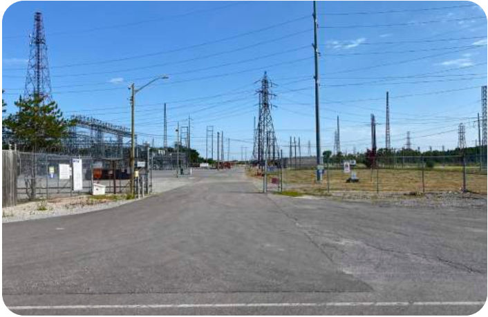
1210 Barron Road, Hydro One Allanburg Transmission Station. View looking north.
