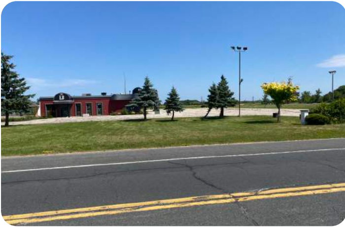
View of Subject Site. Looking South.
