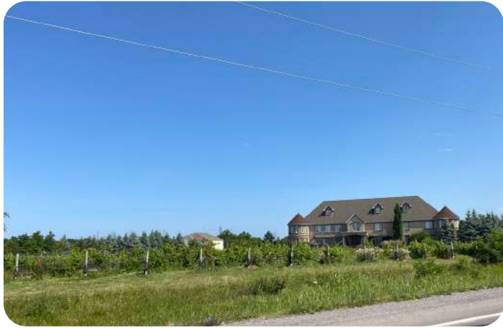
9941 Lundy's Lane, also known as Lundy Manor Wine Cellars. View looking north.
