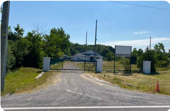
6200 Thorold Townline Road, also known as Heritage Event Centre. View looking east.
