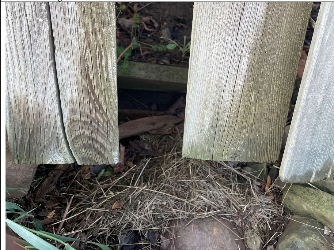
Photo 2: Existing Concrete CB Box Visible Through Existing Fence
