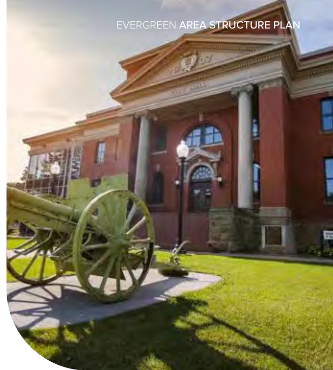
City of Wetaskiwin City Hall
